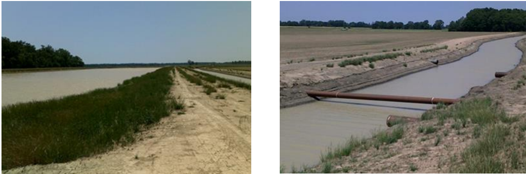
Figure 2.2 A typical on-farm water storage pond (left) used to store water from a tail water recovery ditch (right).
